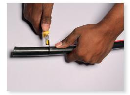
2. Measure the approximate length that will go into the panel and cut off the outer sheathing.
