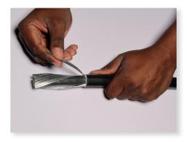
5. Snap-off the armouring from the cable.
