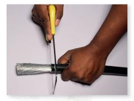
4. Using a junior hacksaw\*, cut the armoring ¾ through making sure you do not damage the inner sheathing.
