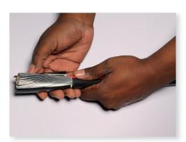
3. Remove the outer sheathing from the cable.
