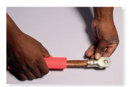
Slide the cut tubing over the object that you're covering; if you'll be splicing, slide the tubing over the centre of the splice, and allow for equal overlap on both sides.
