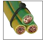
Nylon cable tie tensioned and cut i.e. no sharp edges
