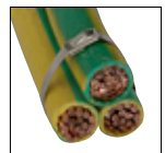
Stainless steel cable tie tensioned/cut/no sharp edges
