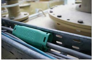
Gel cable joint Relifix V in use as a cable repair.
