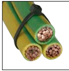
Nylon cable tie tensioned and cut i.e. no sharp edges
