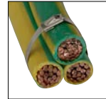
Stainless steel cable tie tensioned and cut i.e. no sharp edges
